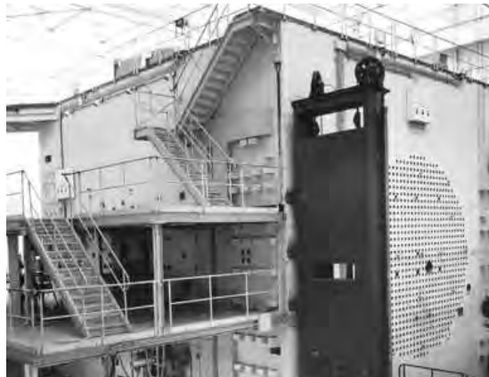
Figure 1.2: The first Belgian Reactor BR1 as of December 1956. The sides A and B with lifting platform for charging the reactor. From [2].
